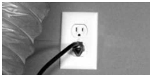
figure 10.2 It is recommended that the HRV or ERV have a dedicated receptacle with 115v. It is not recommended to connect unit with an extension cord. If no receptacle is available please call an electrical contractor and have one installed. Insure polarized is correct
