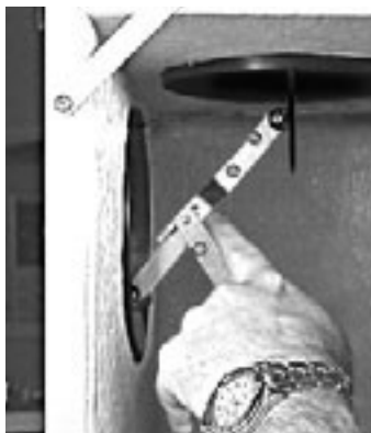
figure 8.2 - Push on the assembly to release the damper
