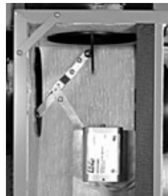
figure 8.3 - Motorized Damper Assembly
