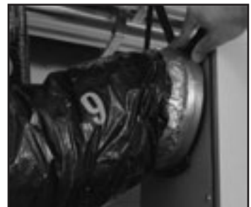
figure 7.4 Slide collar on the unit.
