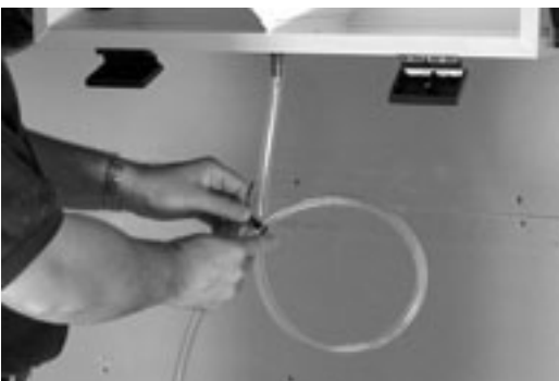
figure 9.1 Make a loop in condensate line, not be subject to freezing temperatures.
