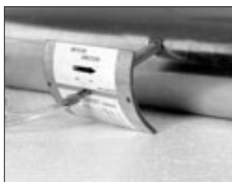
Inserting Air flow grid in duct
